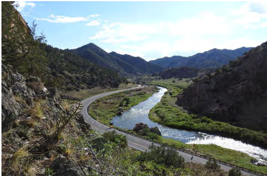
Surface treatment, bridge rehabilitation, and guardrail improvement project on US 50 in Fremont county
