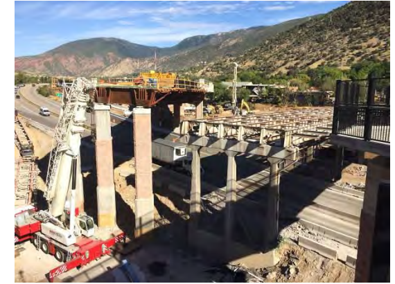
Denver Metro West I-70 Bridges
